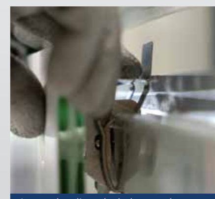
Insert the clip to lock the panel horizontally.
