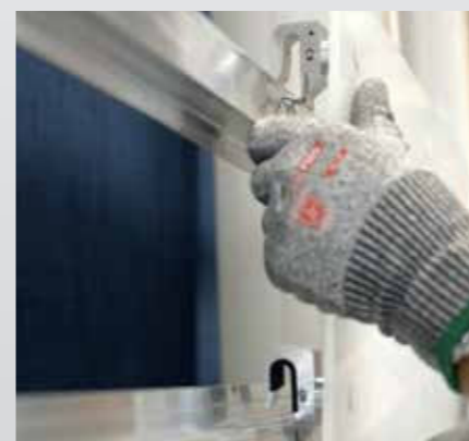
Hang your glass panels on the rails.
